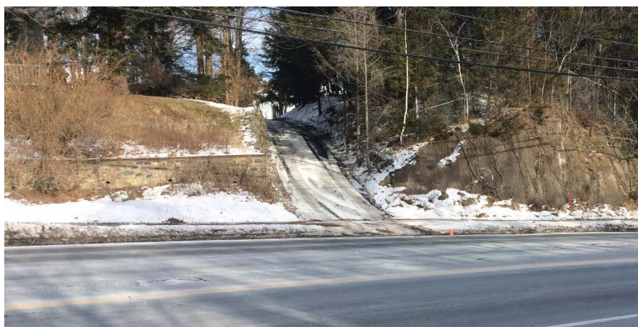
Photo 2: Proposed driveway location at 59 Kearney Lake Road
