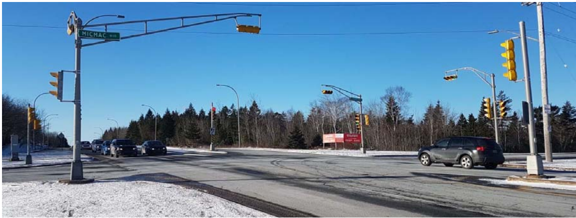
Woodland Avenue at Lancaster Drive/Mic Mac Boulevard looking south
