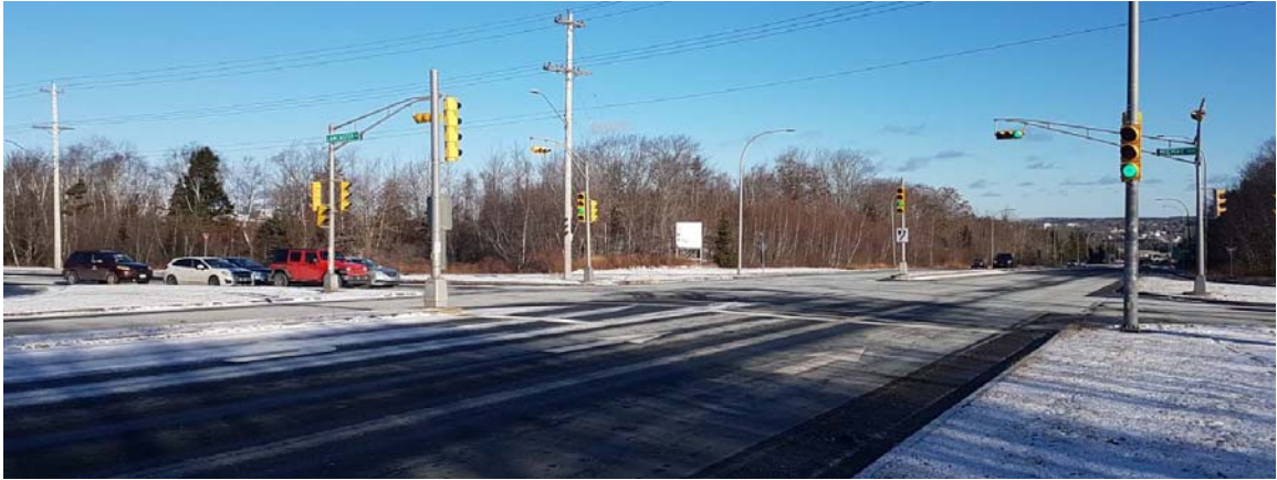
Woodland Avenue at Lancaster Drive/Mic Mac Boulevard looking north
