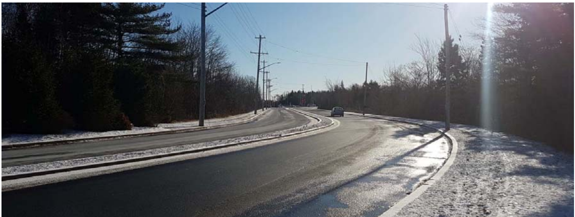
Lancaster Drive at Cannon Terrace/Sea King Drive looking east
