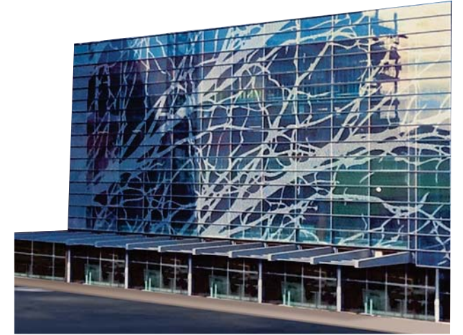
EXEMPLARY PICTURE FROM INTERNET: GLASS CURTAIN WALL IMPRESSIVE DECORATION GLASS CURTAIN WALL WITH CERAMIC PRINT IN TEXAS BY CORGAN
