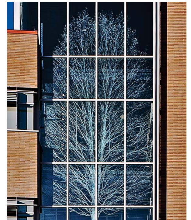
EXEMPLARY PICTURE FROM INTERNET: IMAGES WERE ETCHED ONTO THE GLASS FAÇADE OF LEHIGH UNIVERSITY. SKYLINE DESIGN COLLABORATED WITH BOHLIN CYWINSKI JACKSON ARCHITECTS TO RECREATE TWO ARTWORKS BY LARRY KIRKLAND ON GLASS.
