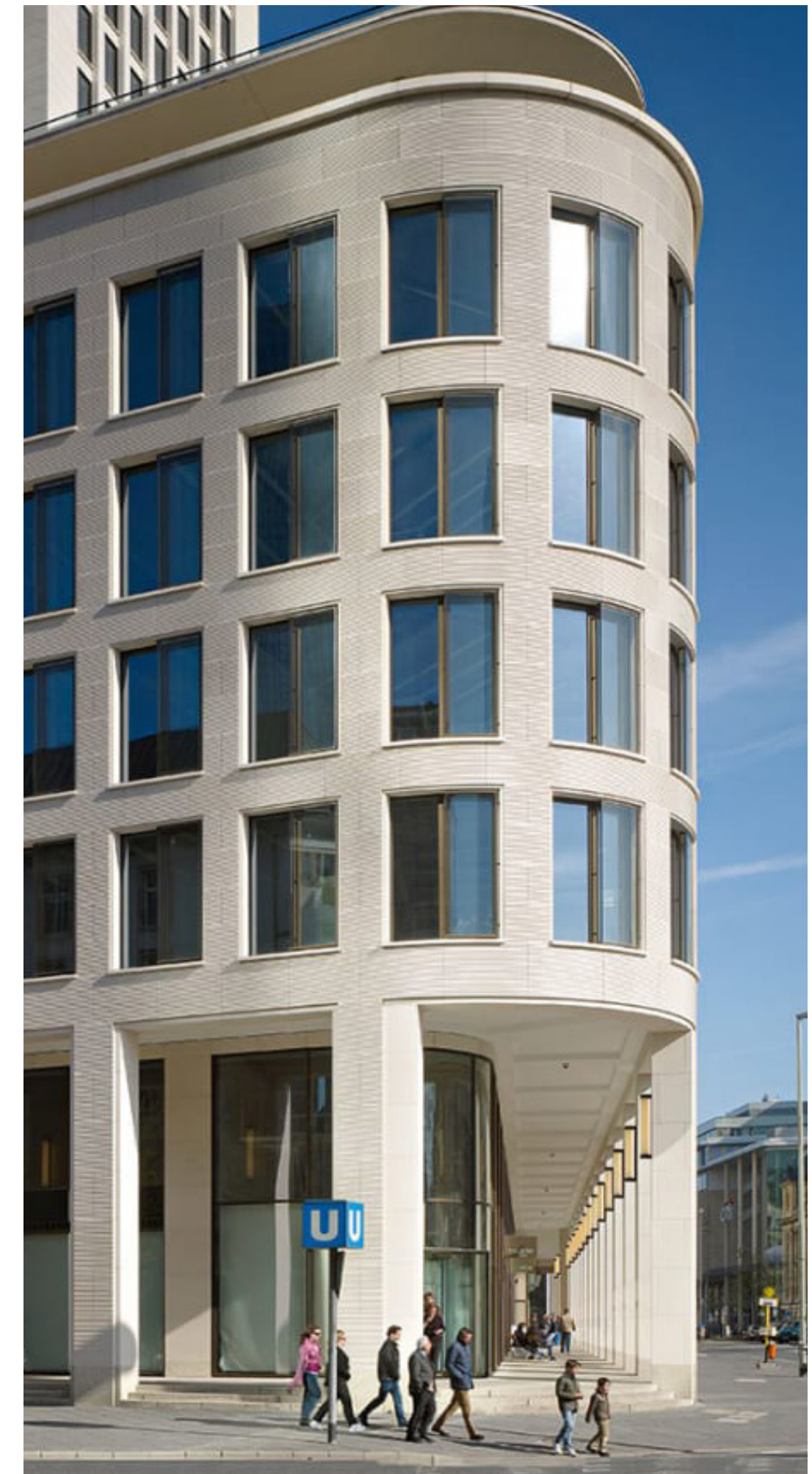
Opernturm, Frankfurt am Main
