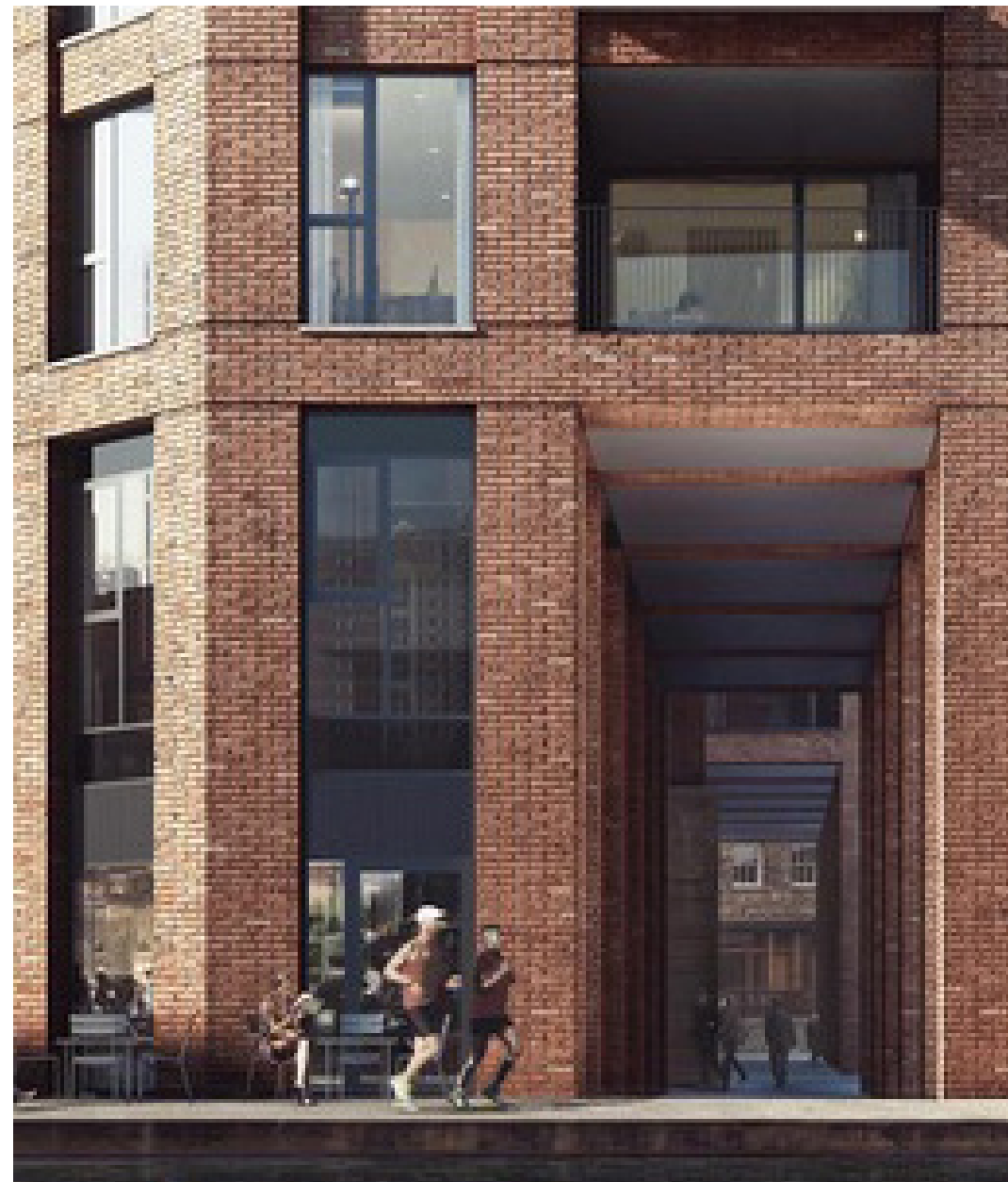
Brick masonry, glass, and feature soffits
