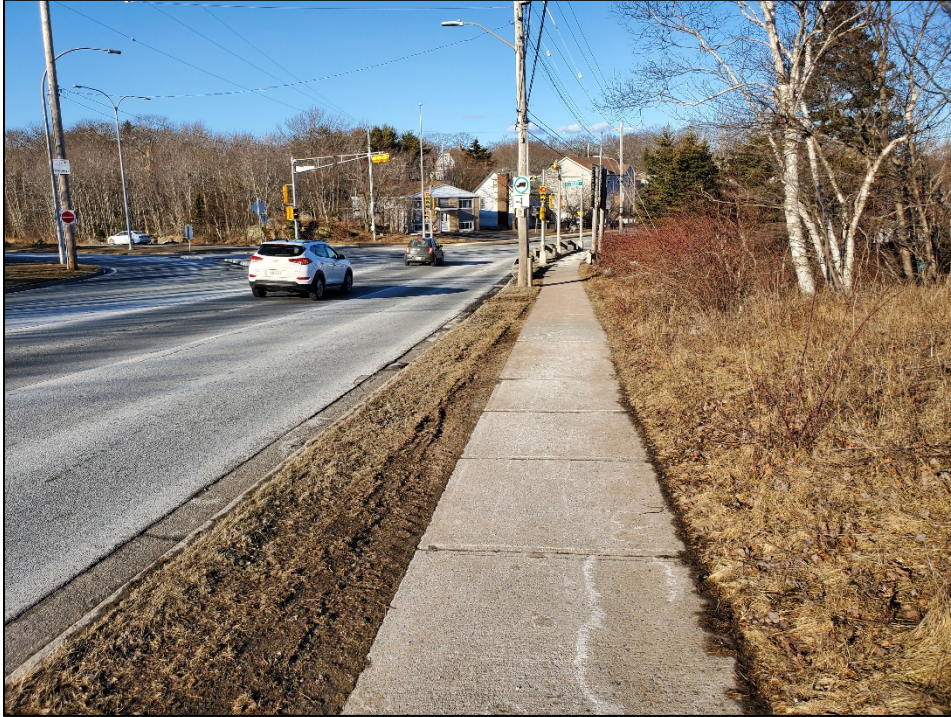
Figure 6: Right View from Access to Old Sambro Road
