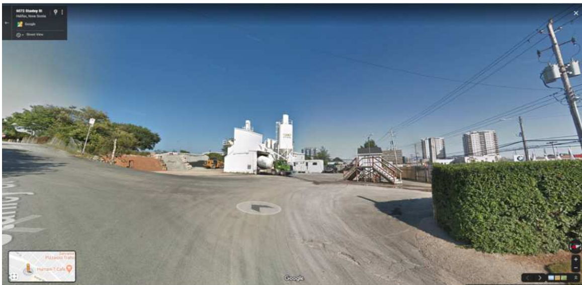
View 1 - Facility view, looking north.
