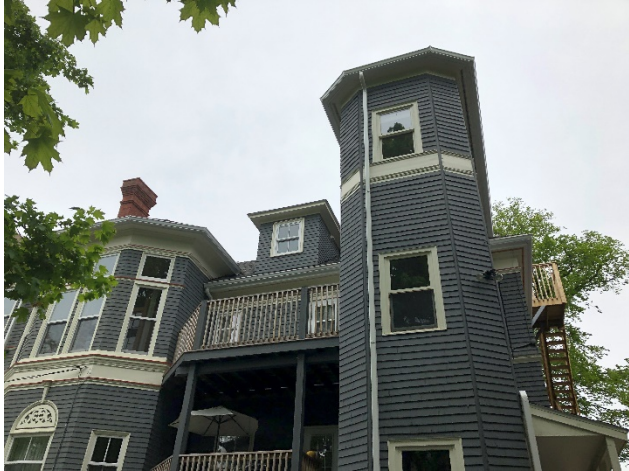
Figure 5: South Side Elevation – Enclosed stair to be removed
