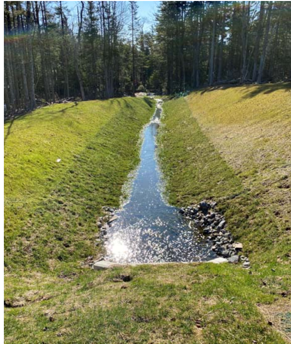
Figure 3.1: Bioswale Outlet, (Parks of West Bedford, Sub-Area 7, 2020)
