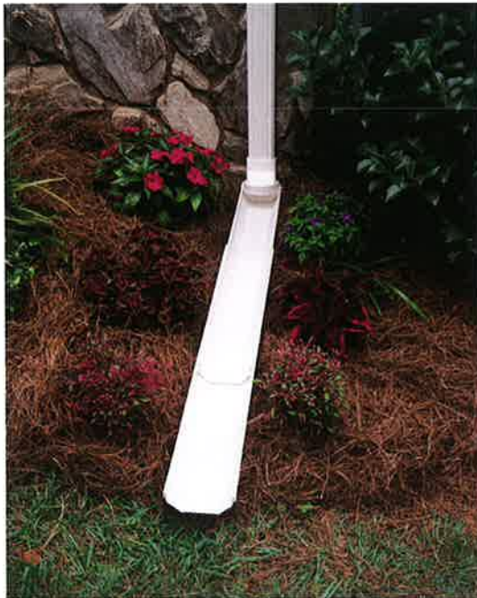
Downspouts should drain the water away from any impervious areas, such as the foundation or driveway, and into vegetated zones.
