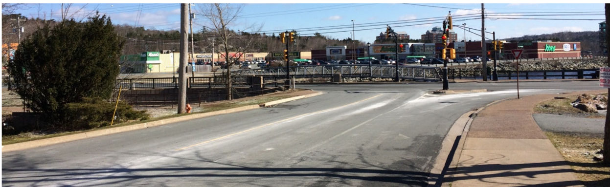
Photo 3 – Looking east on Moirs Mill Road toward the Bedford Highway intersection, the subject site is on the right
