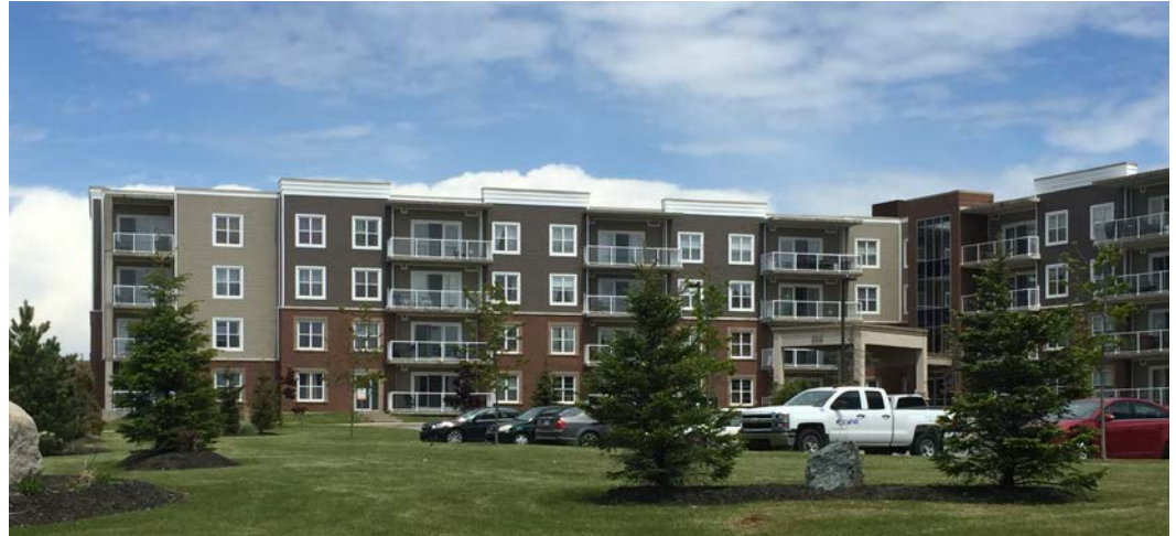
Figure 4: Multi-unit residential building with a small casement windows that are easily accessible from interior of units. First floor units are also raised above grade to improve safety and security
