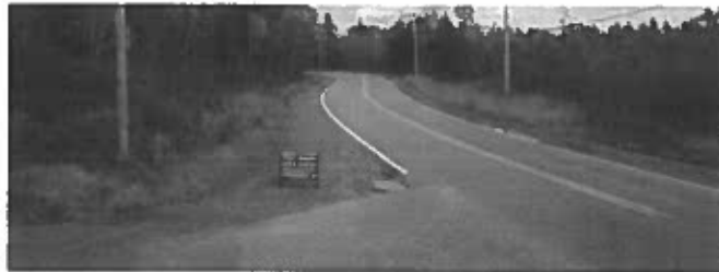
Photo 1 - Looking north on Trunk 2 towards Enfield from the Frenchmans Road Intersection.
