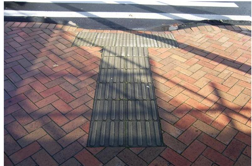
Figure 5: Attention and Directional TWSI's at mid-block crossing (Source: Global Alliance on Accessible Technologies and Environments)
