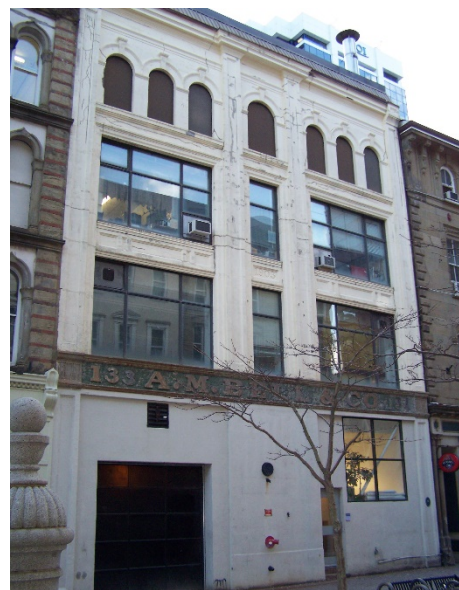
Figure 2: A.M. Bell Building, 2009 Source: HRM Property Files
