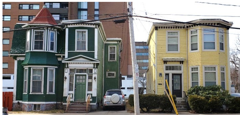
Figure 2: 1538 and 1540 Carlton Street in early spring 2020
