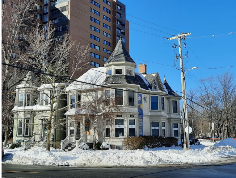
Figure 17: 5945 Spring Garden Road and 5943 Spring Garden Road, with the former locations of 1538 and 1540 Carlton Street visible to the right (09 February 2021)
