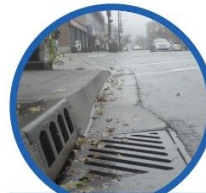
Storm Drains (Catchbasins)
