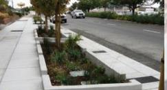
**5** The bicycle lane buffer can double as a series of rain gardens, treating and cooling stormwater while providing aesthetic benefit.
