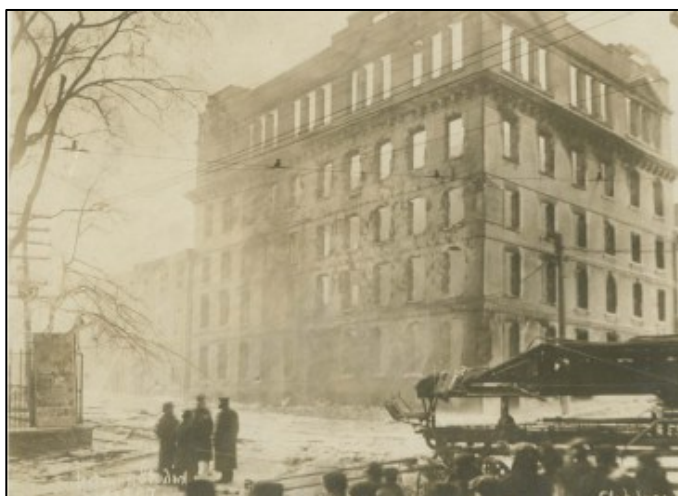
Figure 6: The Kenny-Dennis building showing the shell of the four-storey granite façade topped by the one-storey 1901 addition, shortly after the fire in 1912. Source: NSARM
