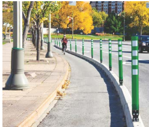
Figure 8: Example of Durable, Flexible Bollards in Ottawa, ON
