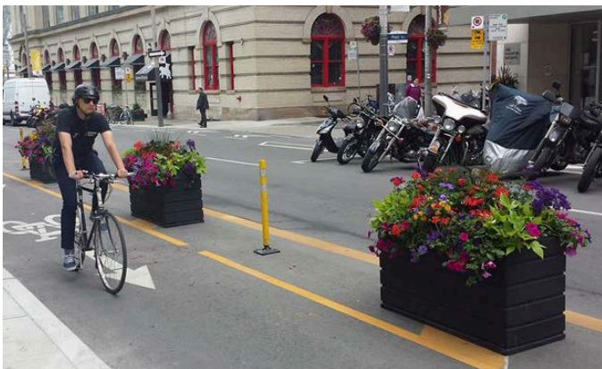
Figure 9: Example of Planter Boxes as Physical Separation for Bicycle Lane in Toronto, ON
