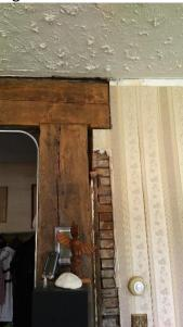
Figure 4: Wall Replaced with Post and Beam
