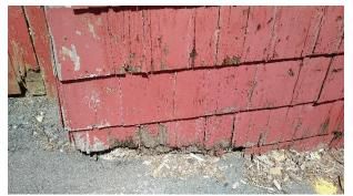
Figure 1: Deteriorated Siding
