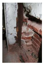
Rusting on embedded structural columns due to moisture penetration through the masonry Source: CMEL
