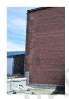
Northwest corner deterioration, significant cracking in the wall assembly Source: CMEL
