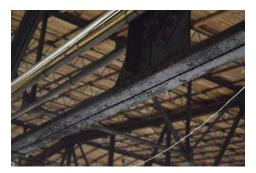
Rust and paint bubbling on truss members Source: CMEL
