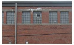
Facade condition, efflorescence and glass block windows Source: CMEL
