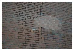
Brick deterioration and inappropriate repairs Source: CMFL
