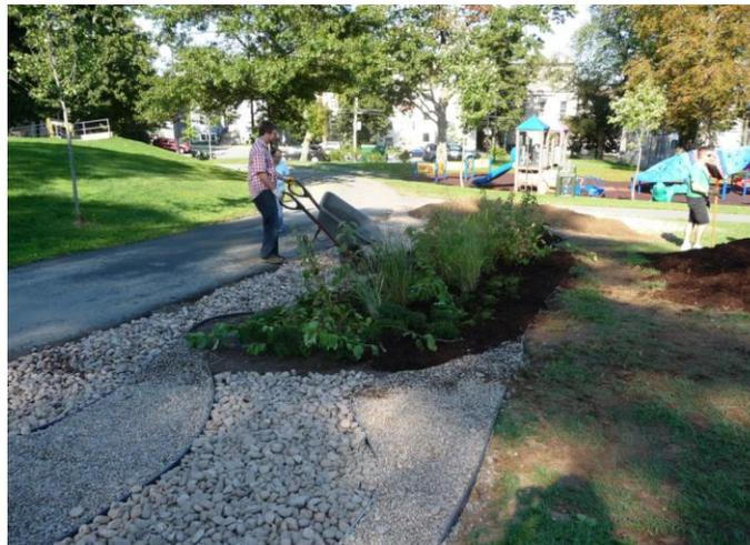
Figure 4 - A rain garden being constructed outside the George Dixon Center in Halifax, with the help of the Ecology Action Center
