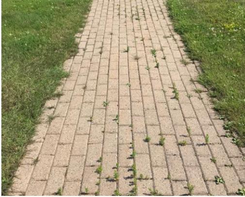
Figure 6 - Permeable pavers in Dartmouth; water can infiltrate between the blocks to a gravel bed below.
