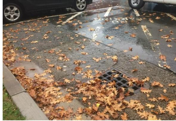
Figure 7 – Porous asphalt in Halifax; water can infiltrate through the asphalt, but sediment may be trapped.
