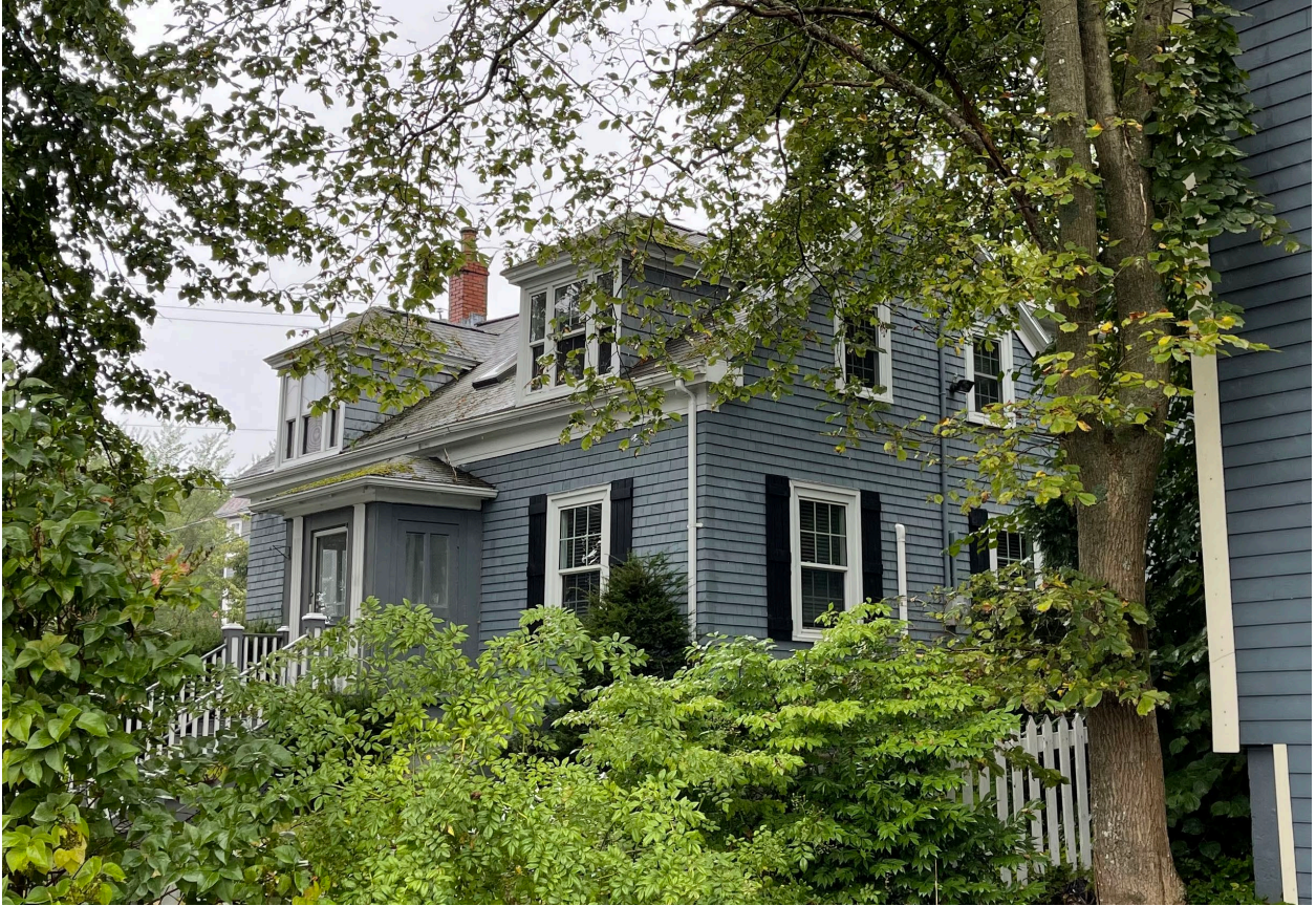
Figure 16: Eastern elevation of 1262 Bedford Highway (August 30, 2021)
