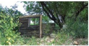
The character-defining elements of Doukhobor Dugout House NHSC in Saskatchewan, such as the window frames, had suffered visible deterioration from exposure to the elements. A long-term repair solution was necessary to prevent further decay and to preserve the site's heritage value.
