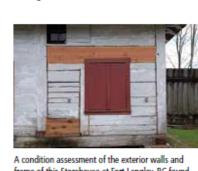
A condition assessment of the exterior walls and frame of this Storehouse at Fort Langley, BC found extensive deterioration of some timbers, which required replacement in kind. The dimensions, hewn finish and species of wood used in the repairs matched those replaced. The photograph shows part of one storehouse wall after the repairs were completed, but before the new timbers were whitewashed.
