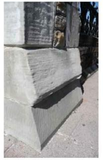
The new pieces of stone on the Wellington Wall at the Parliament Grounds in Ottawa are clearly visible on close inspection due to a different tooling technique.
