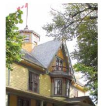
When the windows of Lefurgey House in Summerside, PEI were damaged in a fire, instead of replacing the entire windows, only the broken glass was replaced. The replacement glass, salvaged from a nearby house that was replacing its windows, had similar properties and wavy appearance.
