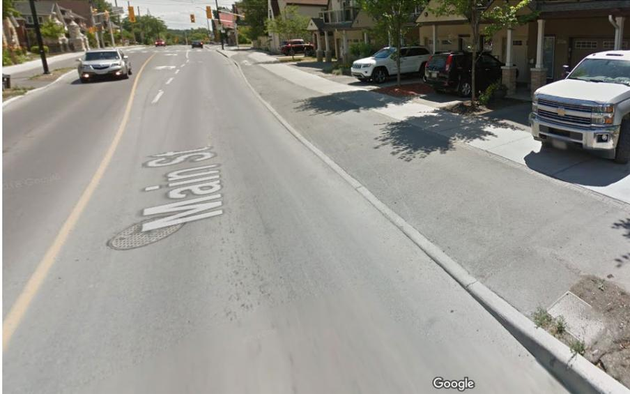
Figure 8 - Example of a continuous driveway apron treatment in Ottawa, ON (from Google Maps)
