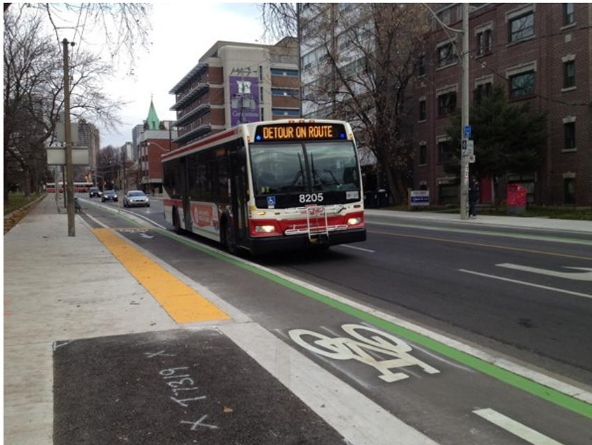
Figure 17 - Transit stop adjacent to a raised cycle track, where cyclists must stop for transit passengers in Toronto, ON (from The Urban Country)
