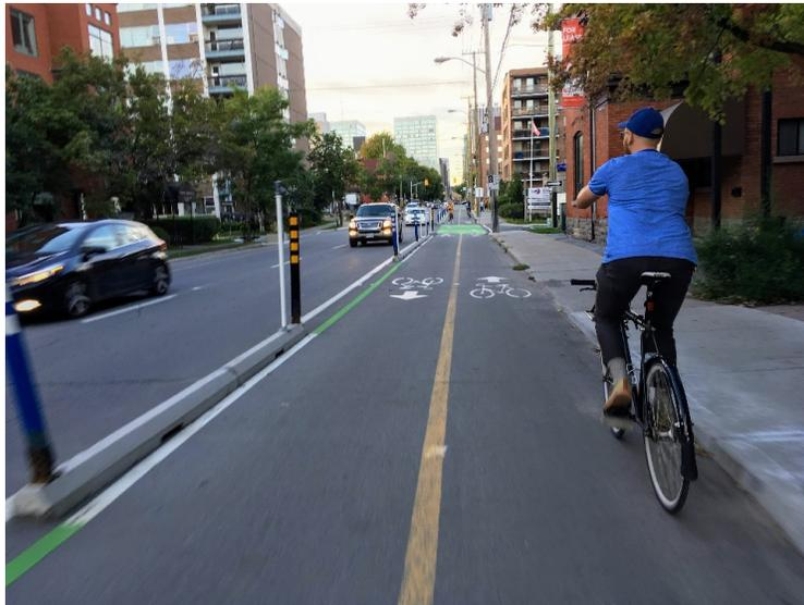
Figure 9 - An example of precast concrete curbs separating an on-road protected bicycle facility in Ottawa, ON
