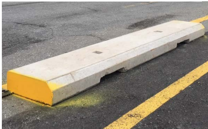
Figure 7: Pre-cast Concrete Curb Prototype Developed for South Park Street Bicycle Lanes
