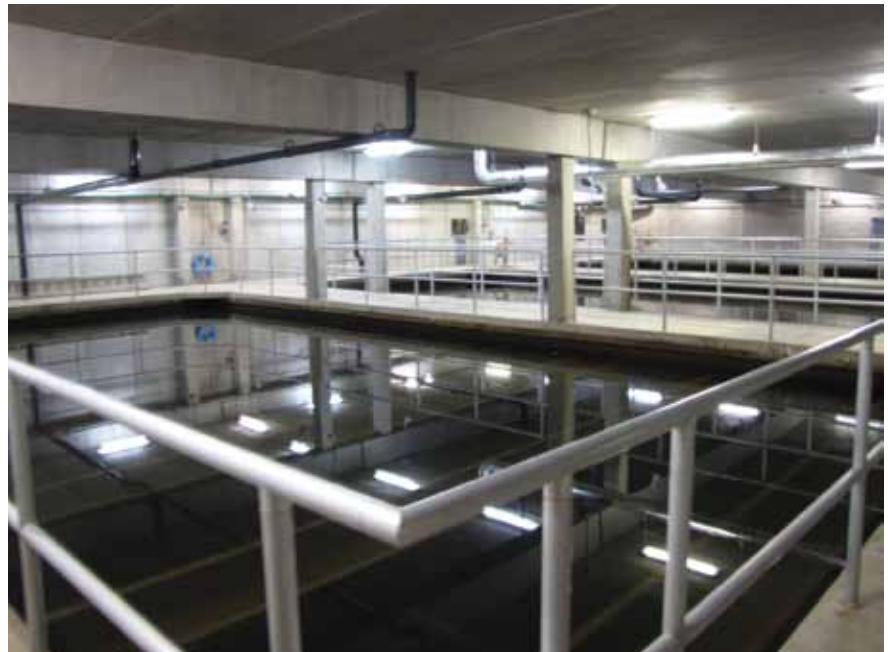
Pockwock water treatment facility, filter gallery
