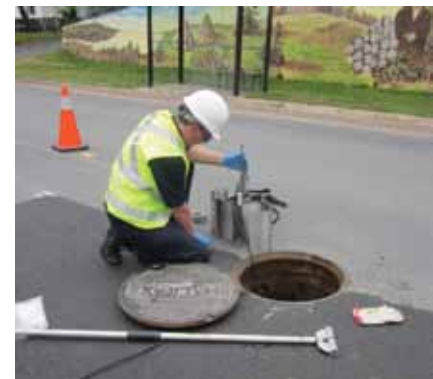
Environmental Engineering staff install a flow meter to monitor stormwater discharge to the wastewater system.
