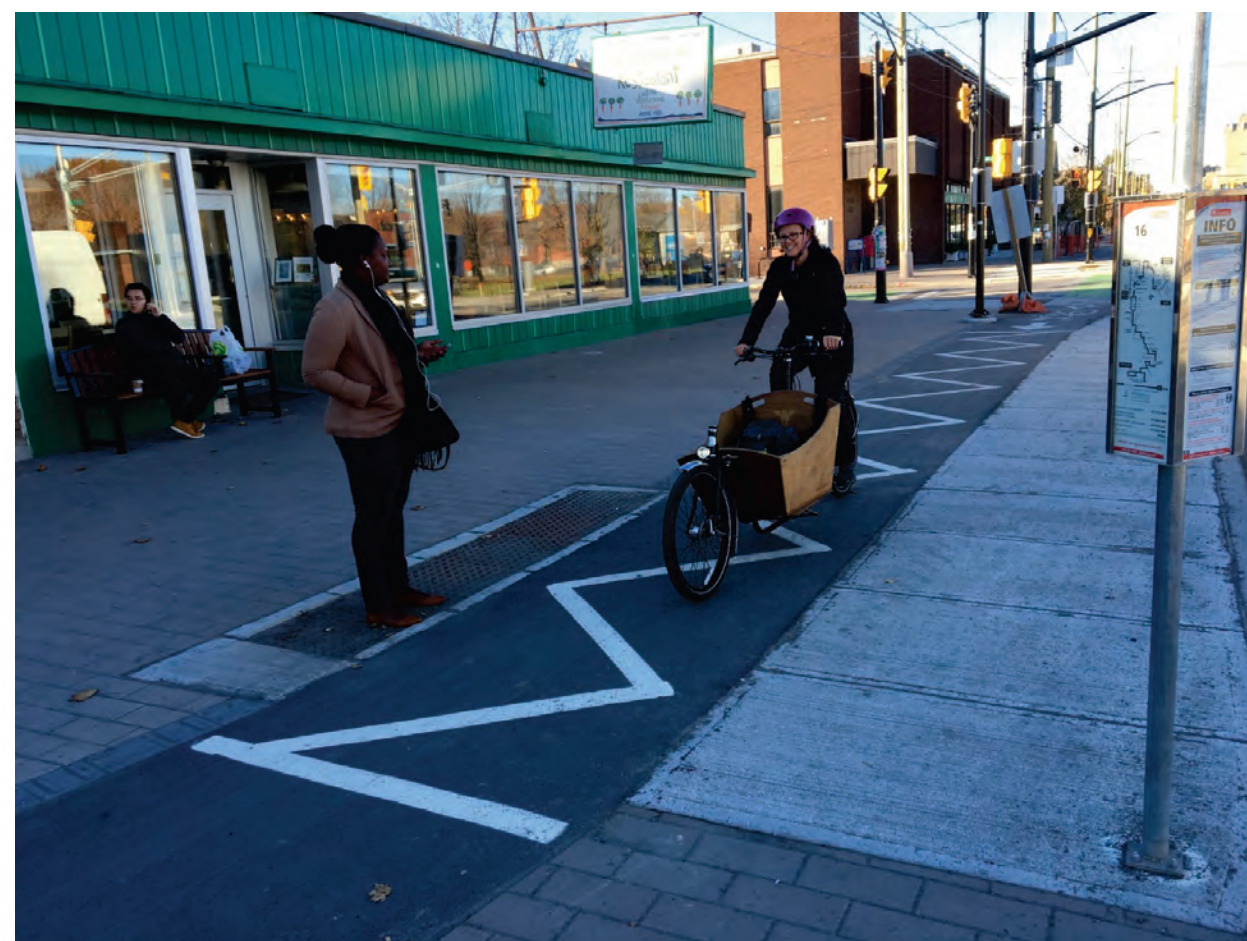
Example of Bus Stop with Bike Lane / Cycle Track (Ottawa):
