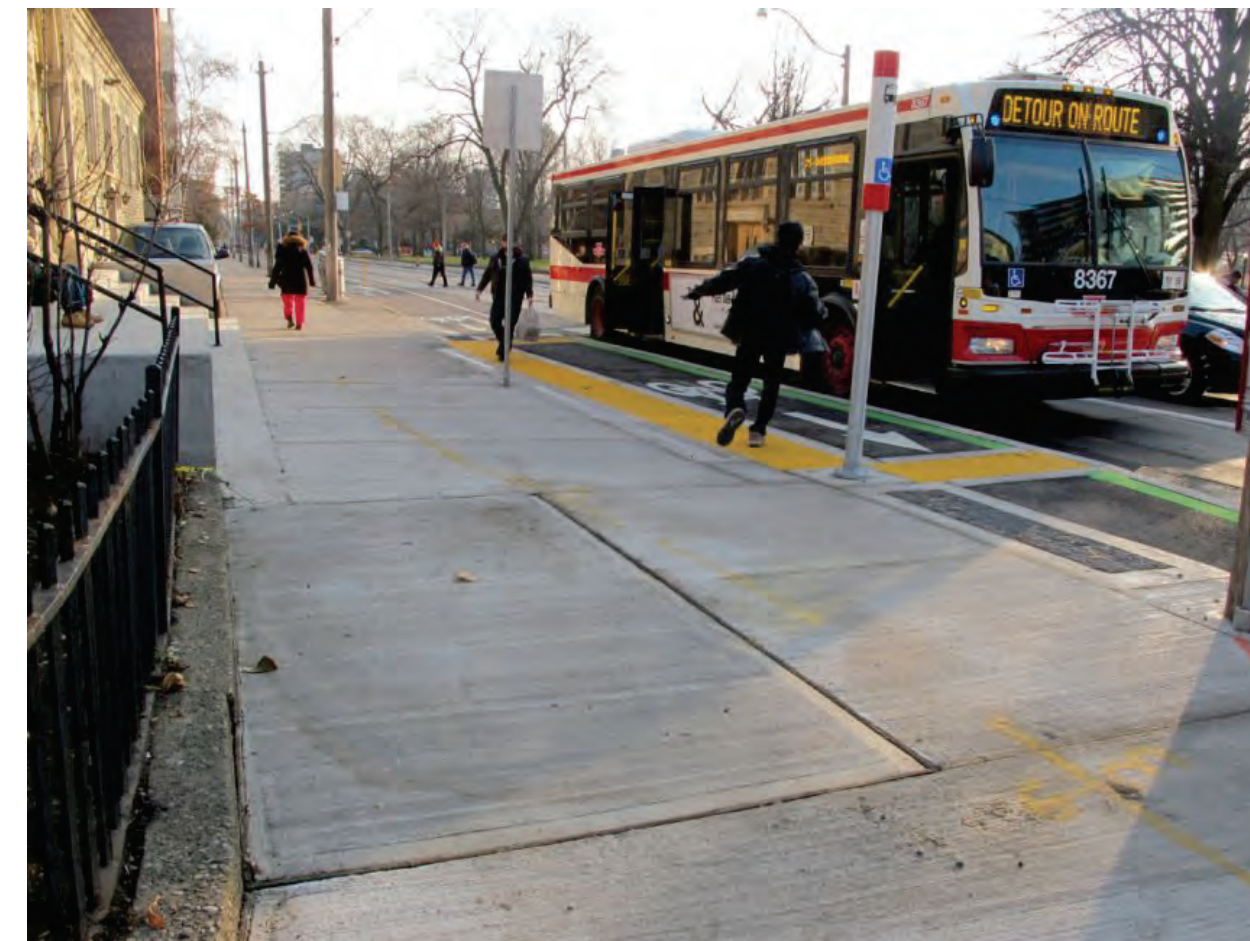
Example of Bus Stop with Bike Lane / Cycle Track (Toronto):
