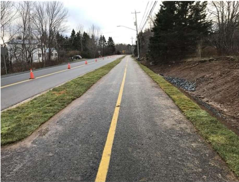
East Preston Greenway- completed in 2024
