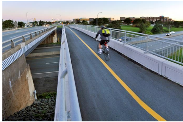
AT Bridge over Hwy 111 at Burnside Dr.
