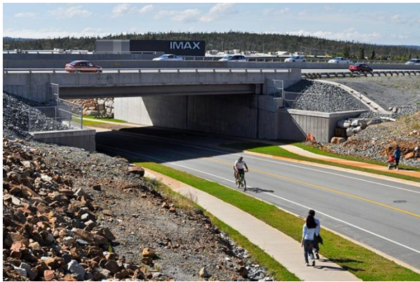
Washmill Lake Road Underpass
