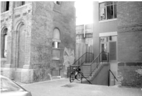
Under-utilized corner adjacent to NFB Building (1998)
