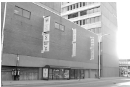
Existing transit stop in front of Scotia Square Mall
