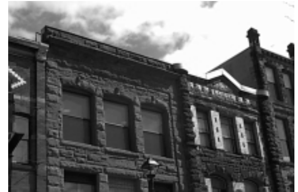
Cabot Building and Kaizer Building
