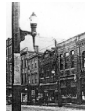
Barrington Street light fixture (circa 1935).
